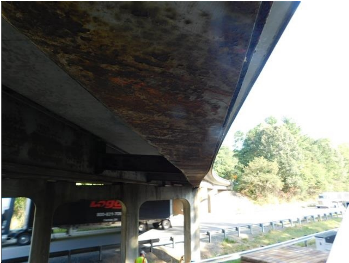
Span 2 Beam 6: Supplemental Inspection Impact Damage, Span 2 Beam 6 Is Bowed Westward 9 Degrees Out Of Plumb For a Length Of 12 Foot That Begins 11.5 Foot From Bent 1. At The Point of Impact The Weld Connecting The Bottom Flange To The Bottom Stiffener Plate Is Broken For 30 Inches. The Point of Impact (Located 20.5 Foot From Bent 1) Also Has Two Gouges On The Bottom Flange. The First One Is 17 Inches Long X 1 Inch High X 3 Inch Deep. The Second One Is 6 Inch Long X 1/2 Inch High X 2 Inch Deep. (PAR)
