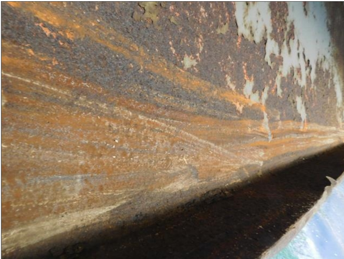
Span 2 Beam 6: Supplemental Inspection Impact Damage 18 Foot Of Scattered Scrapes On Web On The East Side In The Point of Impact Area
