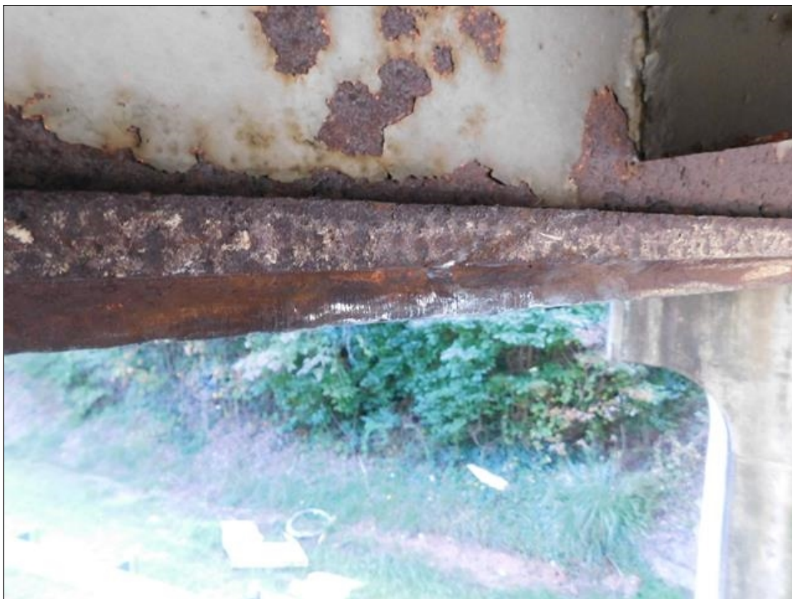
Span 2 Beam 5: Supplemental Inspection Impact Damage Span 2 Beam 5 Has Scattered Scrapes On Bottom Flange On The East Side For 2 Foot Located 15 Foot From Bent 1
