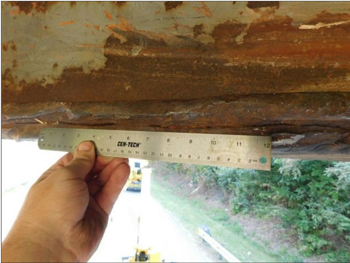
WELD Span 2 Beam 6: Supplemental Inspection Impact Damage, Span 2 Beam 6 Is Bowed Westward 9 Degrees Out Of Plumb For a Length Of 12 Foot That Begins 11.5 Foot From Bent 1. At The Point of Impact The Weld Connecting The Bottom Flange To The Bottom Stiffener Plate Is Broken For 30 Inches. The Point of Impact (Located 20.5 Foot From Bent 1) Also Has Two Gouges On The Bottom Flange. The First One Is 17 Inches Long X 1 Inch High X 3 Inch Deep. The Second One Is 6 Inch Long X 1/2 Inch High X 2 Inch Deep. (PAR)
