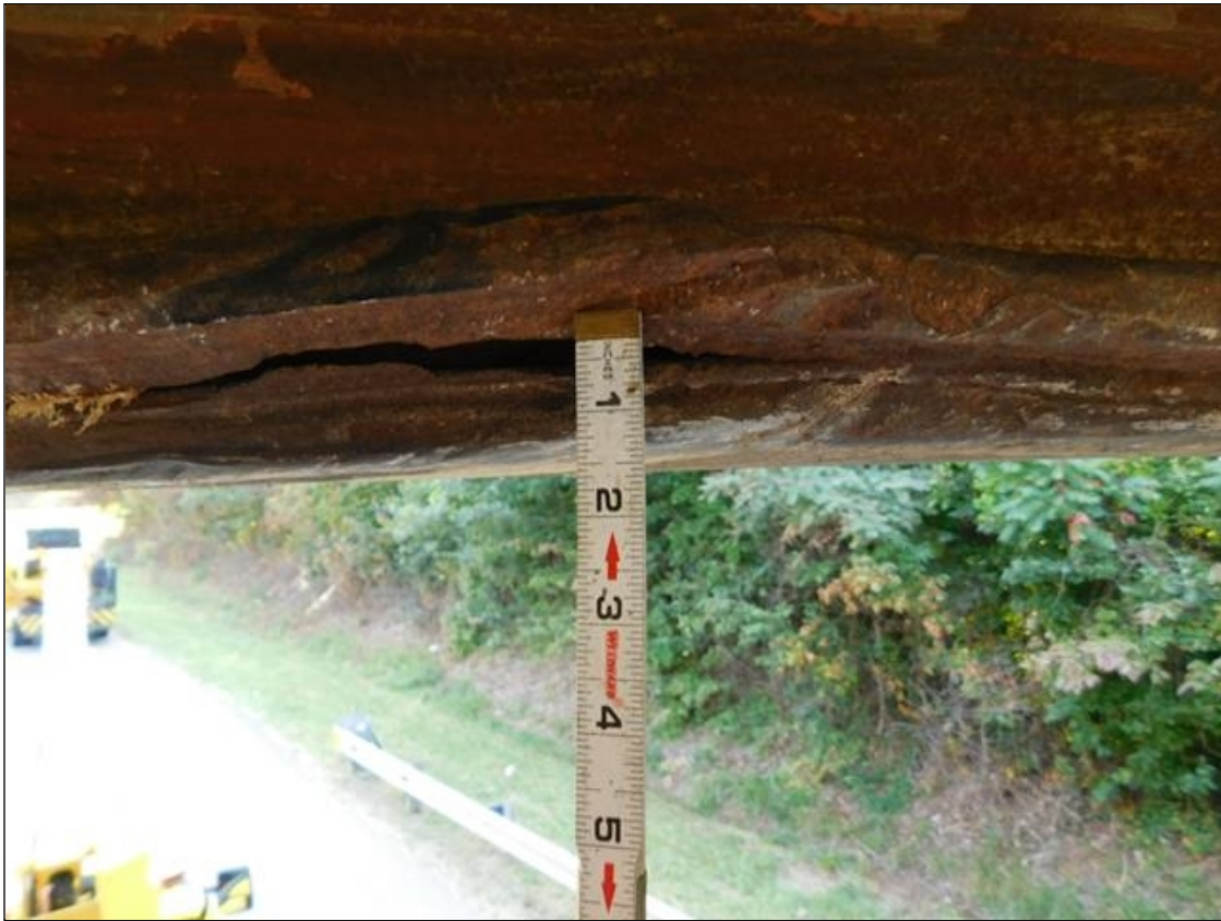
GOUGE ONE Span 2 Beam 6: Supplemental Inspection Impact Damage, Span 2 Beam 6 Is Bowed Westward 9 Degrees Out Of Plumb For a Length Of 12 Foot That Begins 11.5 Foot From Bent 1. At The Point of Impact The Weld Connecting The Bottom Flange To The Bottom Stiffener Plate Is Broken For 30 Inches. The Point of Impact (Located 20.5 Foot From Bent 1) Also Has Two Gouges On The Bottom Flange. The First One Is 17 Inches Long X 1 Inch High X 3 Inch Deep. The Second One Is 6 Inch Long X 1/2 Inch High X 2 Inch Deep. (PAR)
