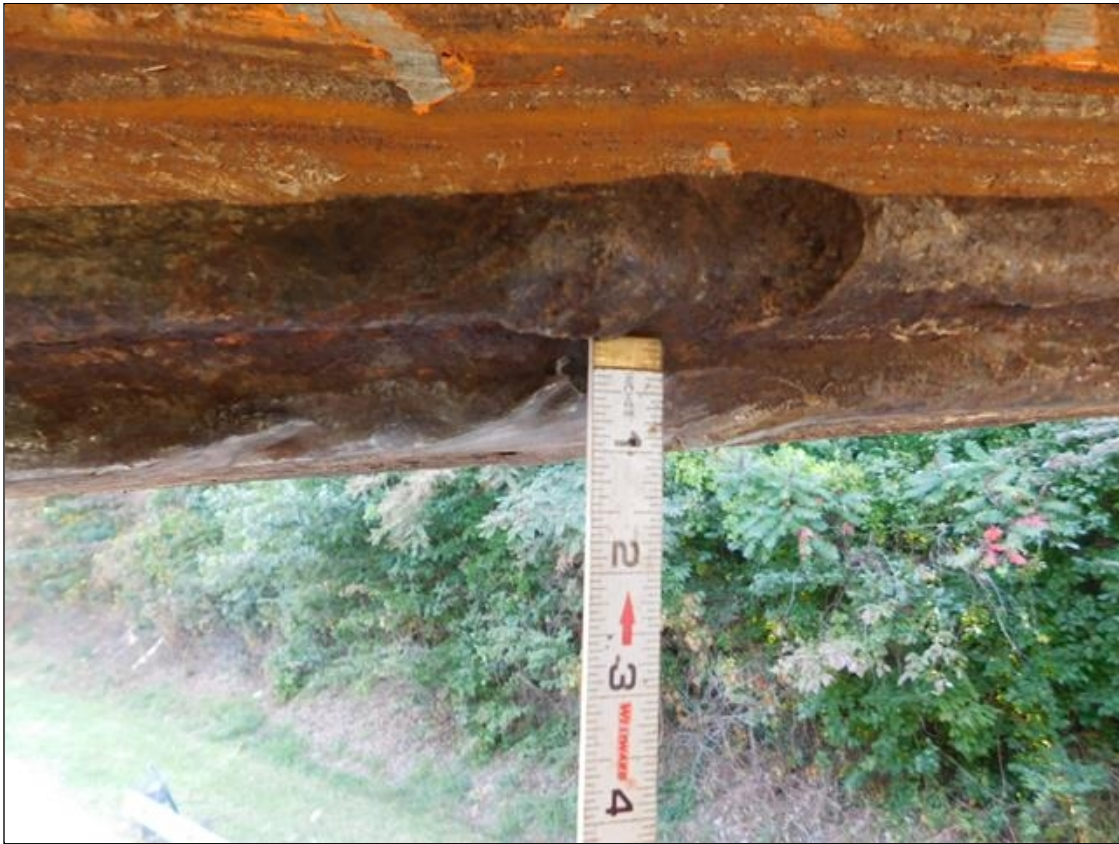
GOUGE TWO Span 2 Beam 6: Supplemental Inspection Impact Damage, Span 2 Beam 6 Is Bowed Westward 9 Degrees Out Of Plumb For a Length Of 12 Foot That Begins 11.5 Foot From Bent 1. At The Point of Impact The Weld Connecting The Bottom Flange To The Bottom Stiffener Plate Is Broken For 30 Inches. The Point of Impact (Located 20.5 Foot From Bent 1) Also Has Two Gouges On The Bottom Flange. The First One Is 17 Inches Long X 1 Inch High X 3 Inch Deep. The Second One Is 6 Inch Long X 1/2 Inch High X 2 Inch Deep. (PAR)
